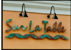
Externally Illuminated Sign
