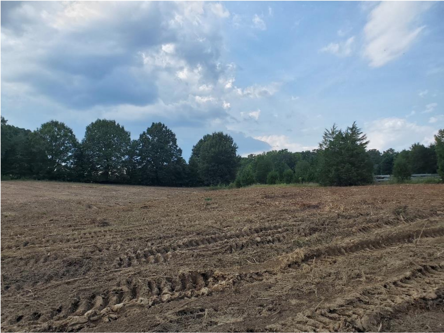
Figure 17: General nature of the land after clearing activity.
