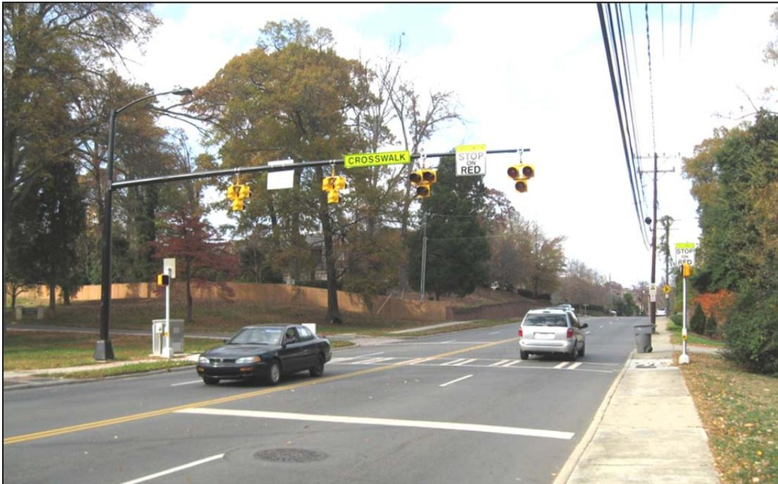
Mid-block crossings with pedestrian actuated signals should be considered when locating these facilities along well-traveled roadways.
