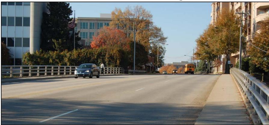
Though most pedestrians prefer separation between sidewalks and travel lanes, bridges often create obstacles for pedestrian travel because of a lack of dedicated facilities. Sidewalks located directly adjacent to travel lanes provide a dedicated facility for pedestrian travel along roadways with lower traffic volumes and speeds.
