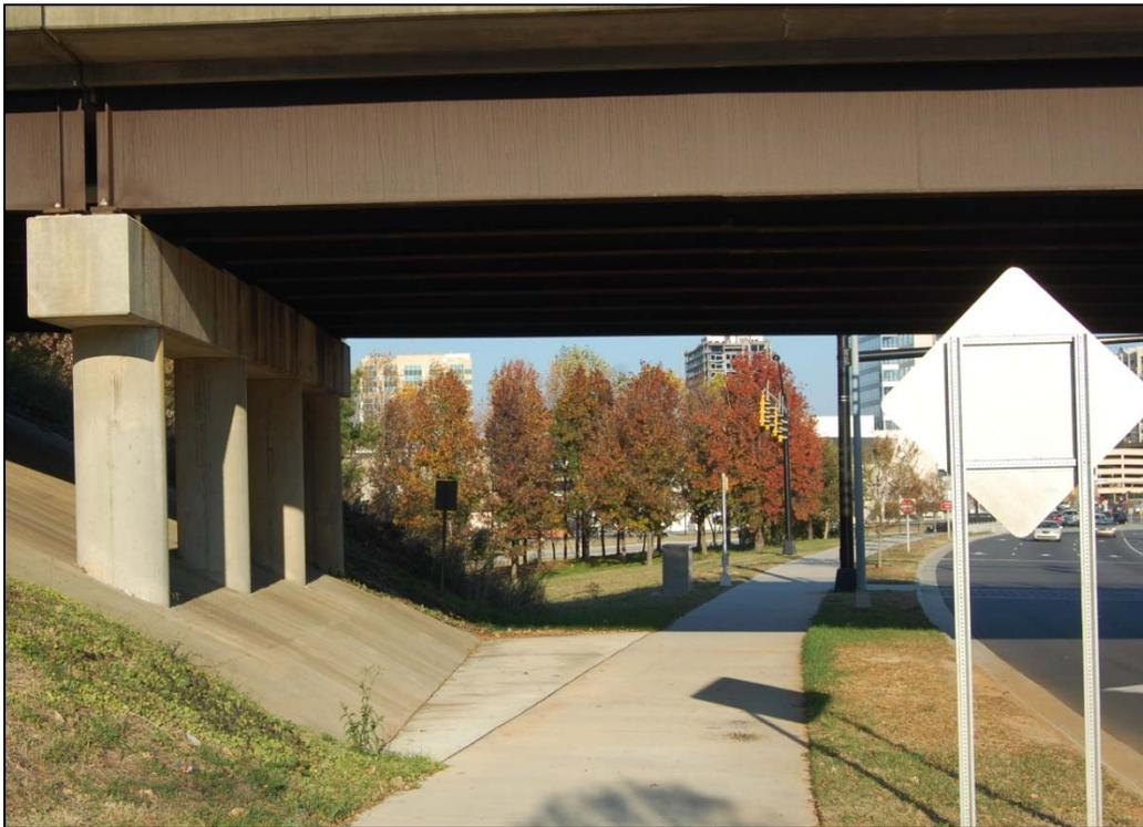
Cyclists and pedestrians have a clear view on both side of the multipurpose path while passing through this underpass. Separation from the travel lanes is also provided.
