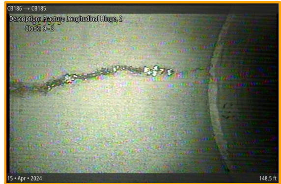
[Grade 3] Fracture Longitudinal Hinge, 2 at 148.5 ft, 9 - 3 o'clock
