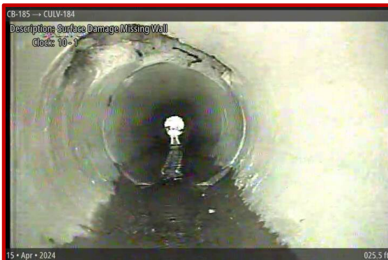
[Grade 5] Surface Damage Missing Wall at 025.5 ft, 10 - 1 o'clock
