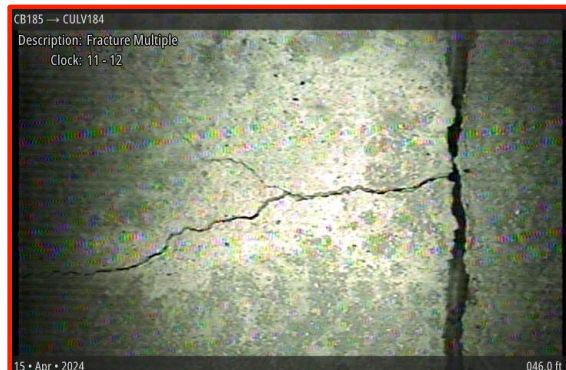
[Grade 4] Fracture Multiple at 046.0 ft, 11 - 12 o'clock
