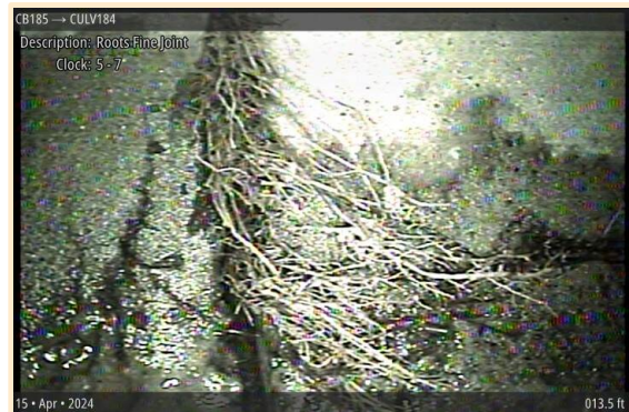
[Grade 1] Roots Fine Joint at 013.5 ft, 5 - 7 o'clock
