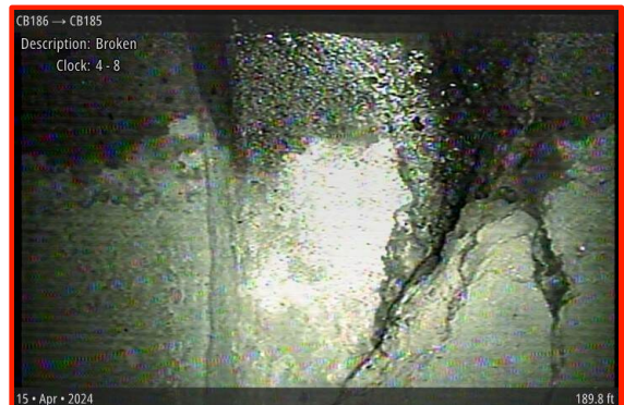
[Grade 4] Broken at 189.8 ft, 4 - 8 o'clock
