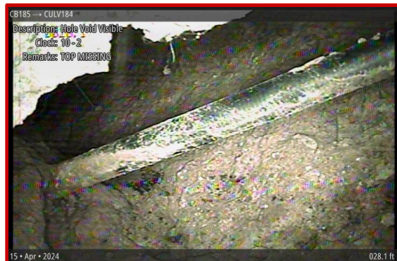
[Grade 5] Hole Void Visible at 028.1 ft, 10 - 2 o'clock | TOP MISSING
