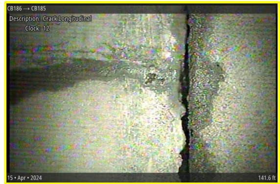
[Grade 2] Crack Longitudinal at 141.6 ft, 12 o'clock
