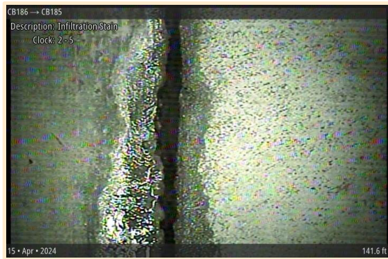
[Grade 1] Infiltration Stain Joint at 141.6 ft, 2 - 5 o'clock
