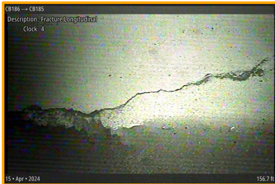
[Grade 3] Fracture Longitudinal at 156.7 ft, 4 o'clock
