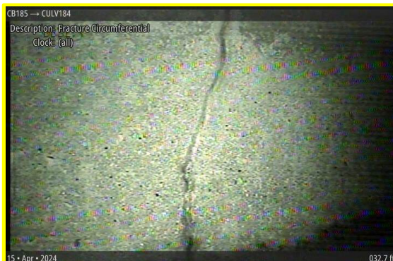
[Grade 2] Fracture Circumferential at 032.7 ft, (all clock positions)
