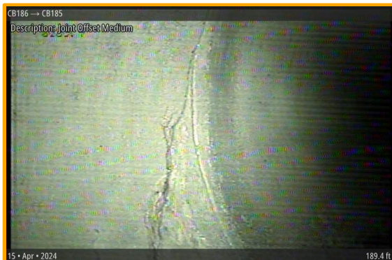
[Grade 3] Joint Offset Medium at 189.3 ft
