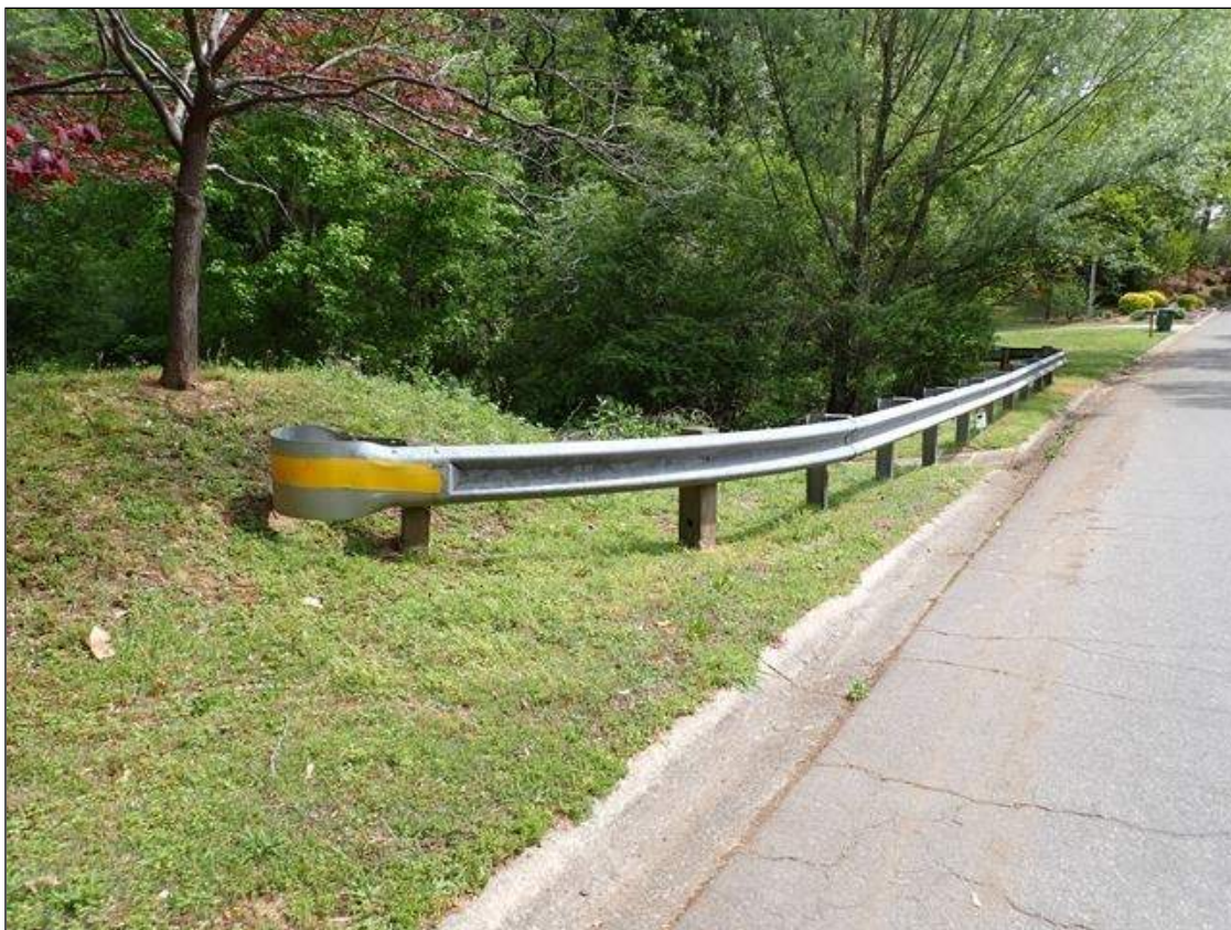
northwest guardrail termination
