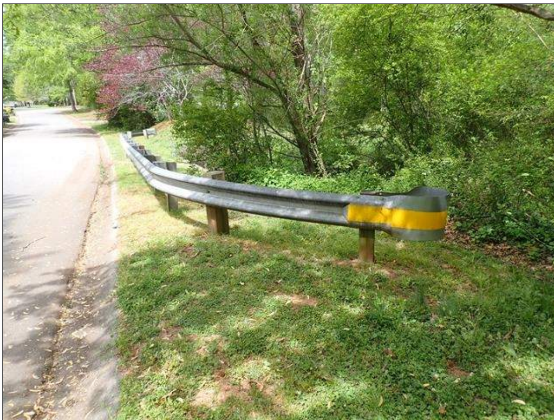
northeast guardrail termination
