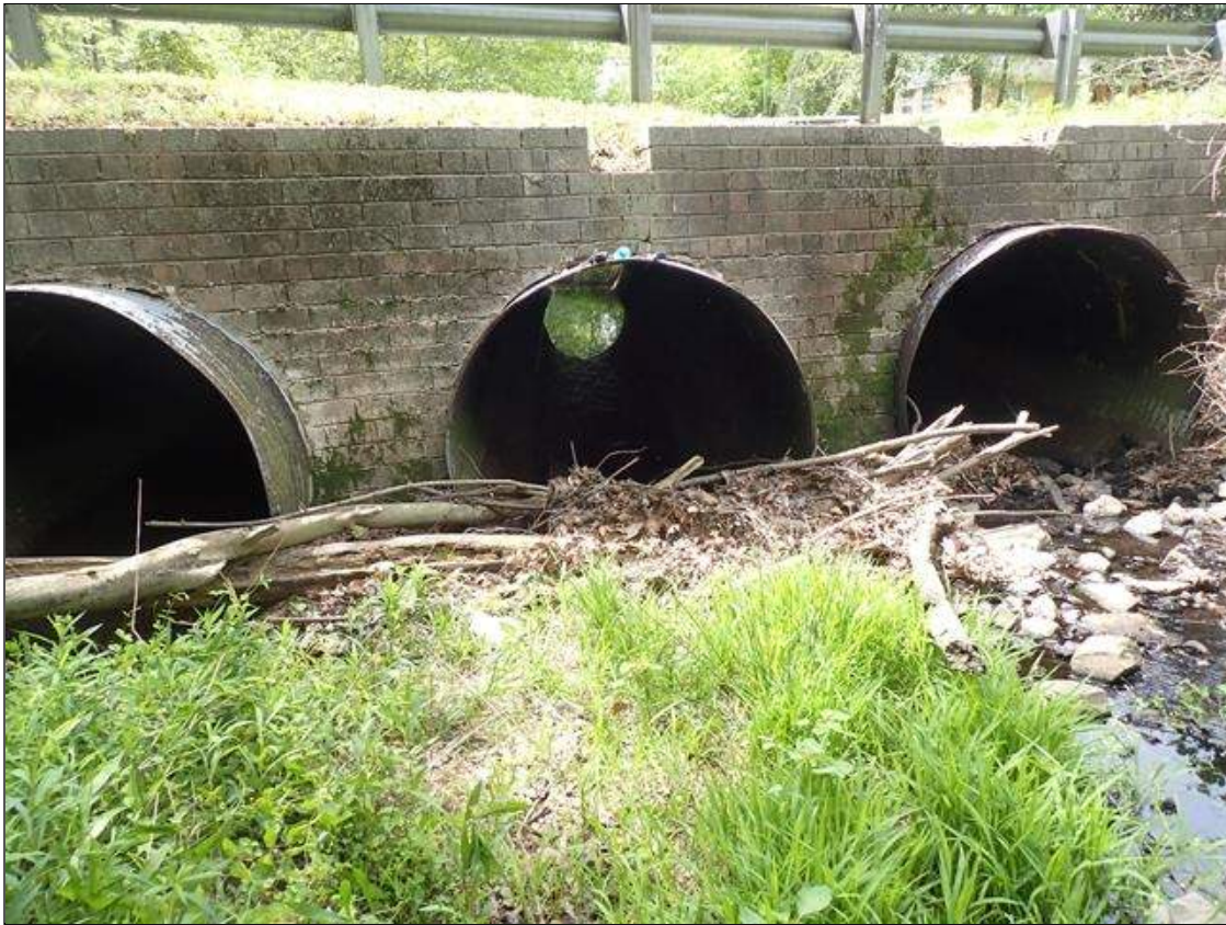
(PAR Municipal) at upstream end, drift partially obstructing flow through barrels
