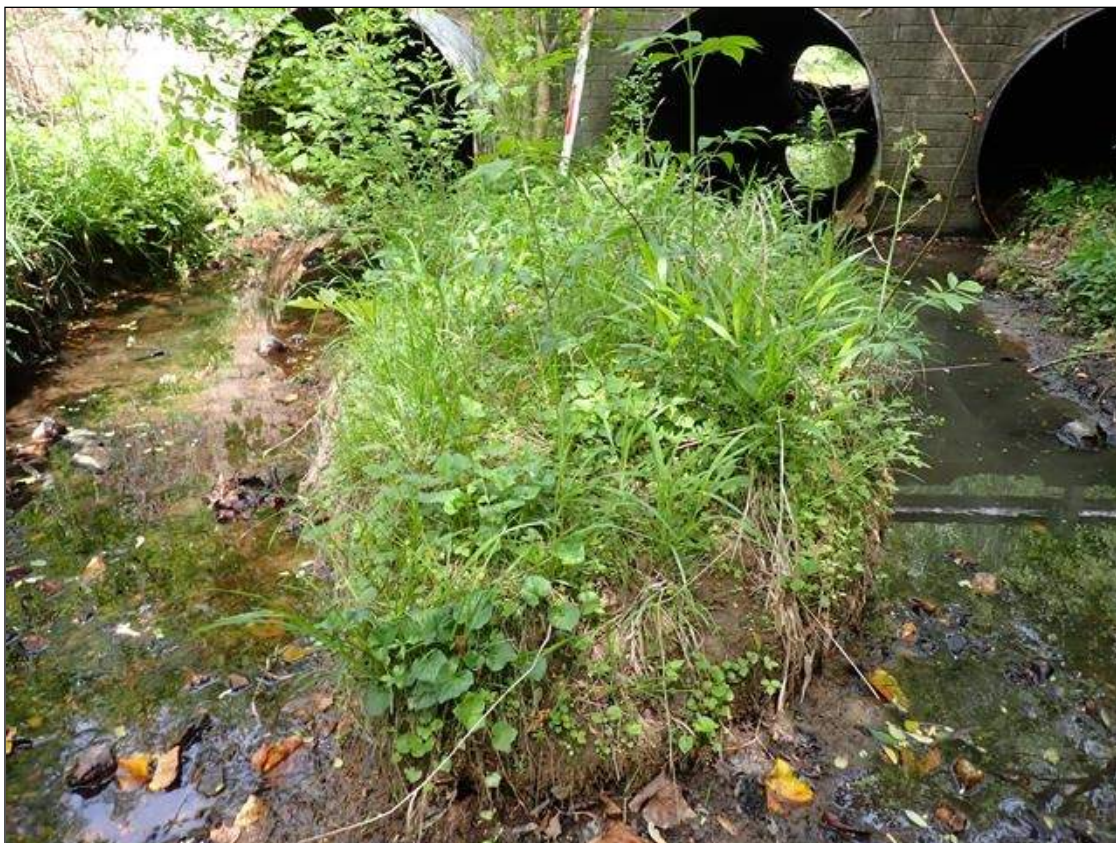
sandbar with vegetation at outlet of barrels 1 and 2 (15 feet x 5 feet x 2.5 feet high)
