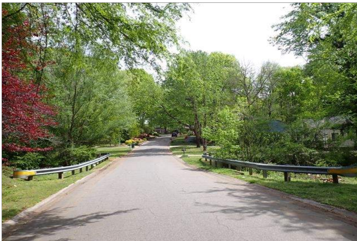
west approach looking east
