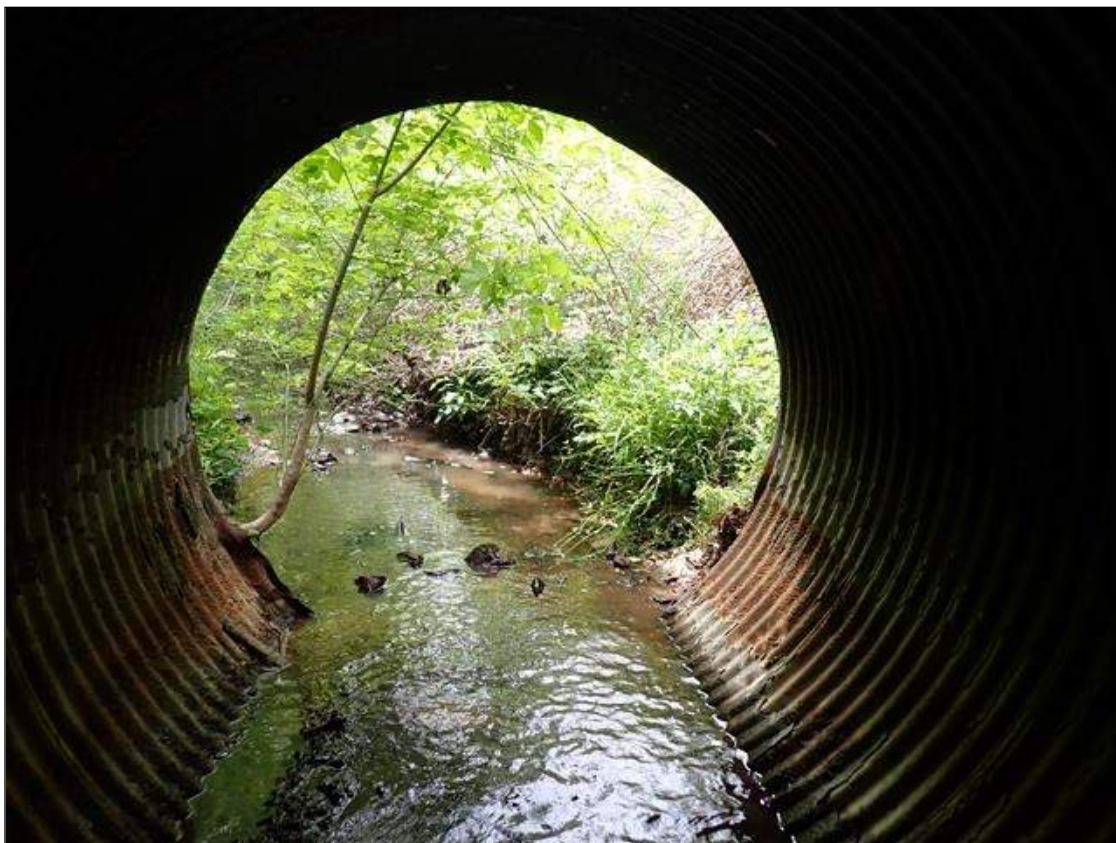
looking downstream from barrel 1
