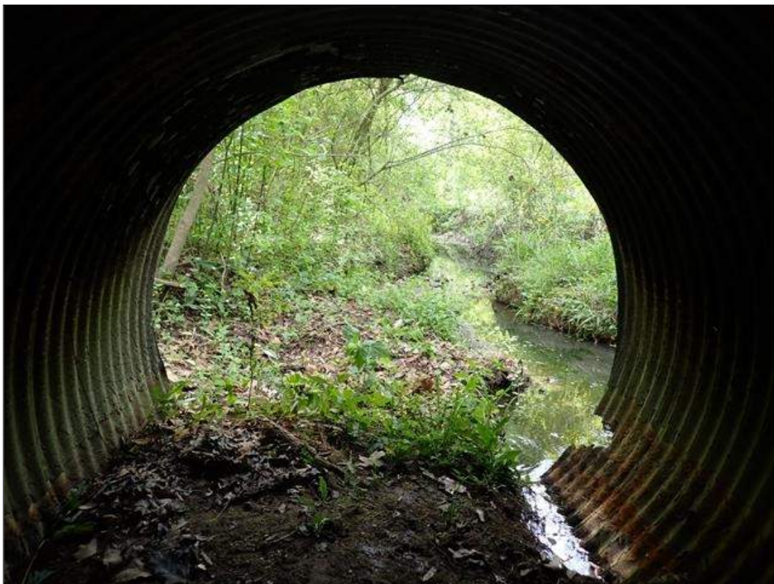
looking downstream from barrel 3
