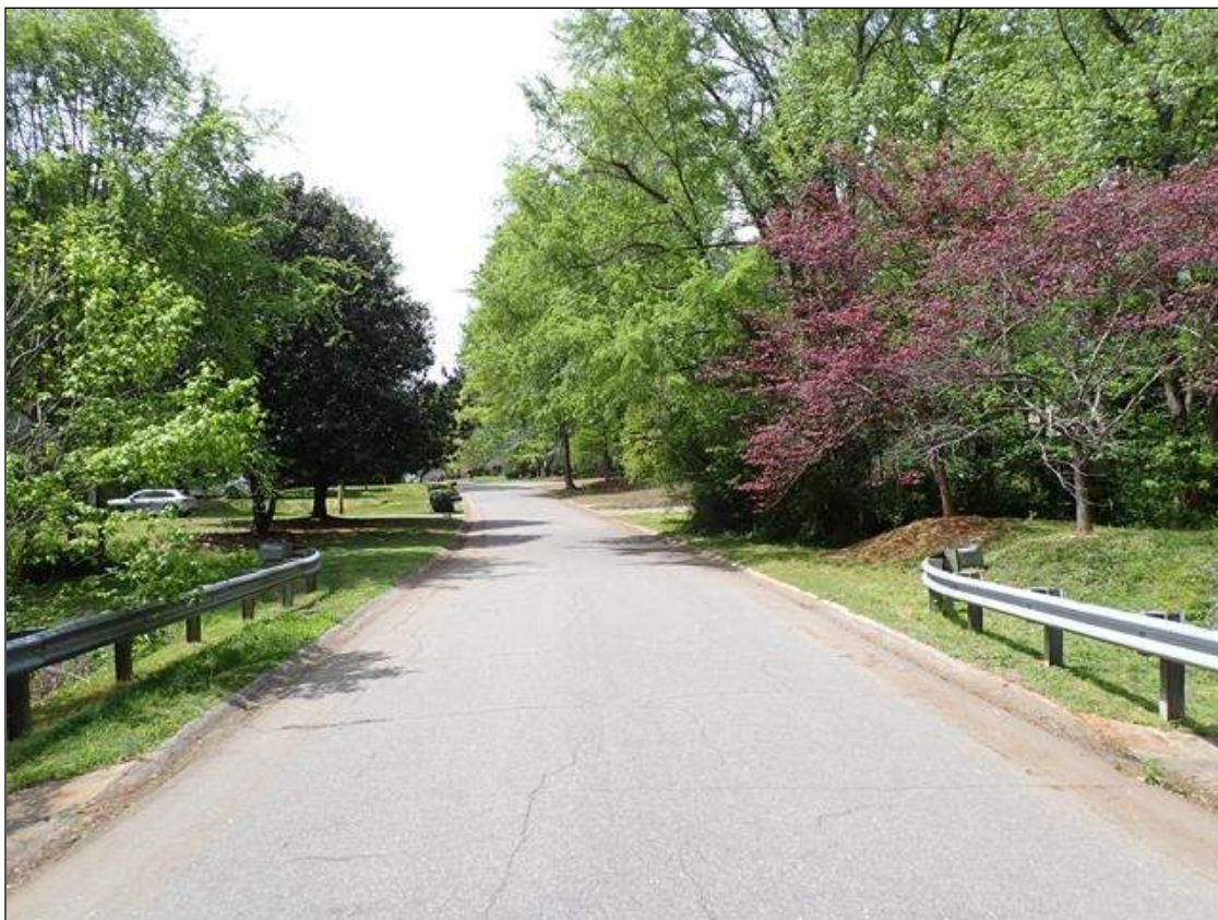
west approach looking west
