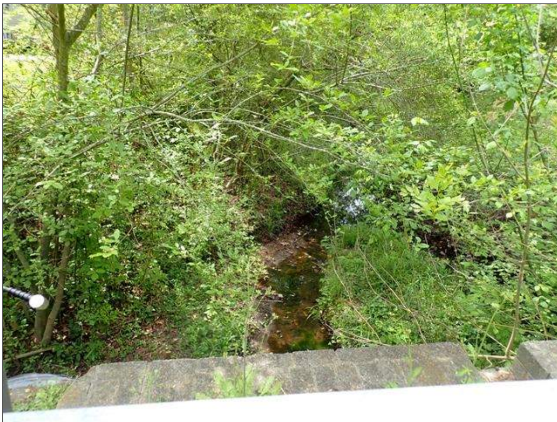
downstream looking south
