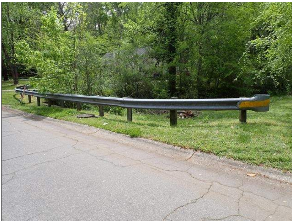
southwest guardrail termination
