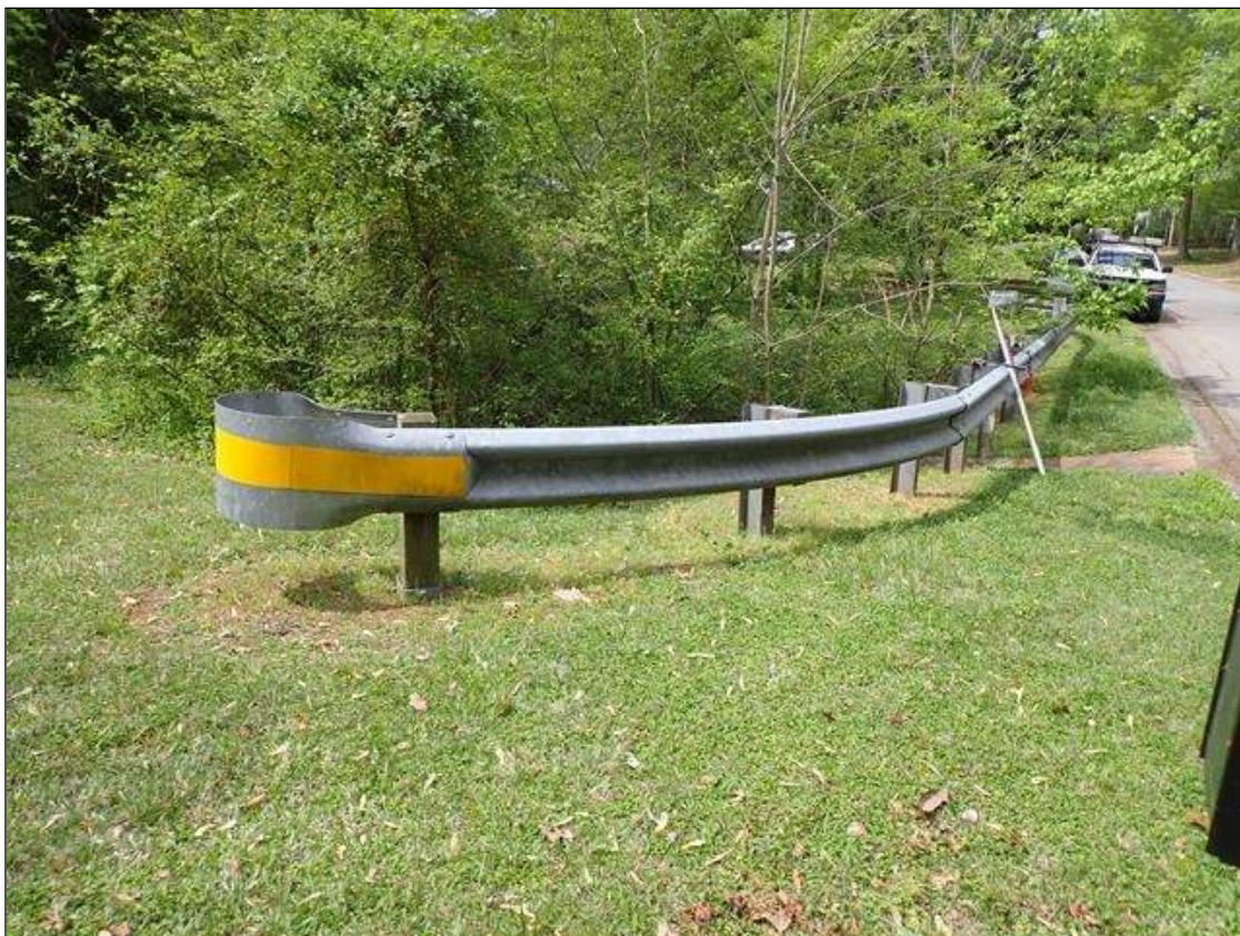
southeast guardrail termination
