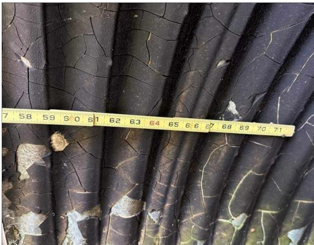
barrel 2 corrugation pattern
