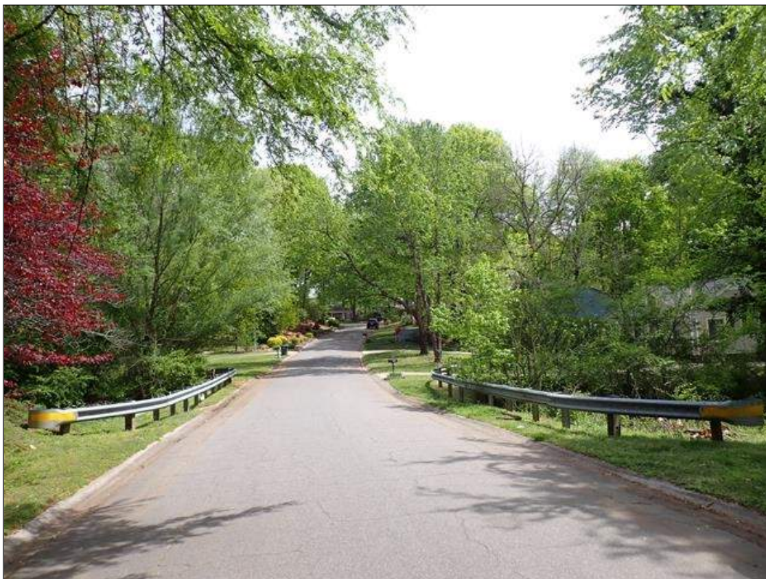
west approach looking east
