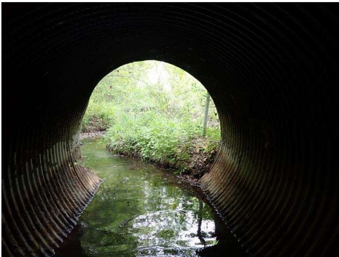
looking downstream from barrel 2
