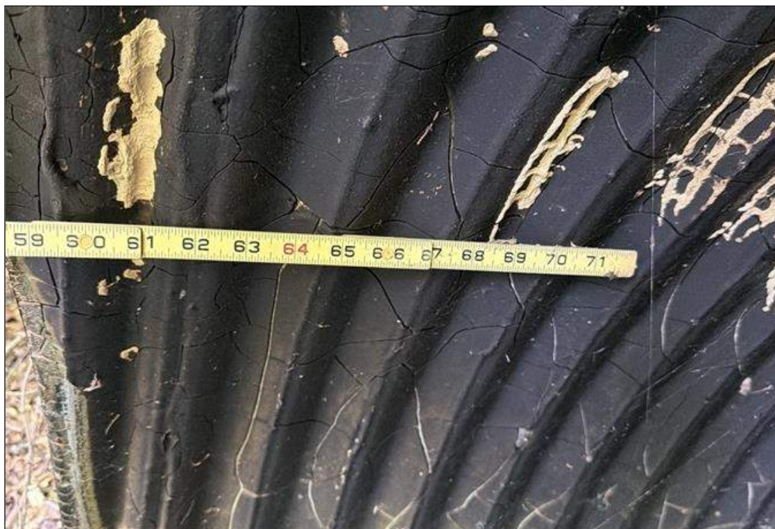
barrel 1 corrugation pattern
